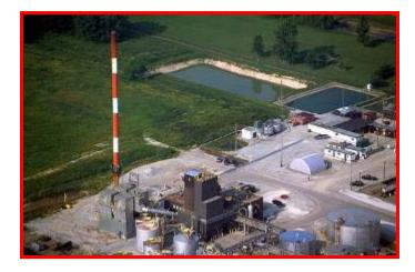
Clean Harbors' Lambton incineration facility is ISO 14001 certified and services Canada and the United States. The facility utilizes a *liquid waste injection incineration* consisting of a fixed unit incinerator, a semi-dry spray dryer absorber, and a four-compartment baghouse. This high-temperature incineration system provides a cost-effective and environmentally sound option for the management of liquid and pumpable materials.
