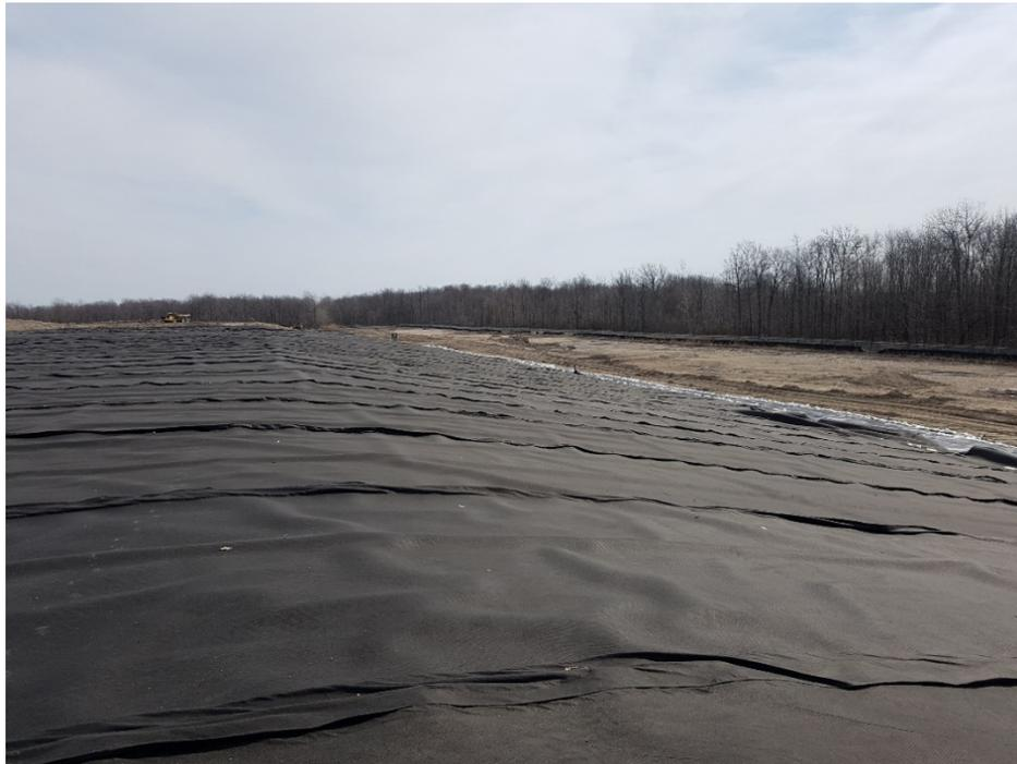
Photo 6 - Final landfill cover placement, Cell 19-1
