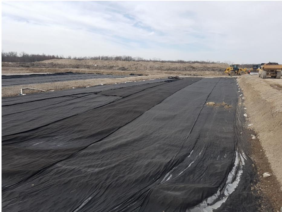
Photo 2 – Completed sub-cells, Cell 19-2
